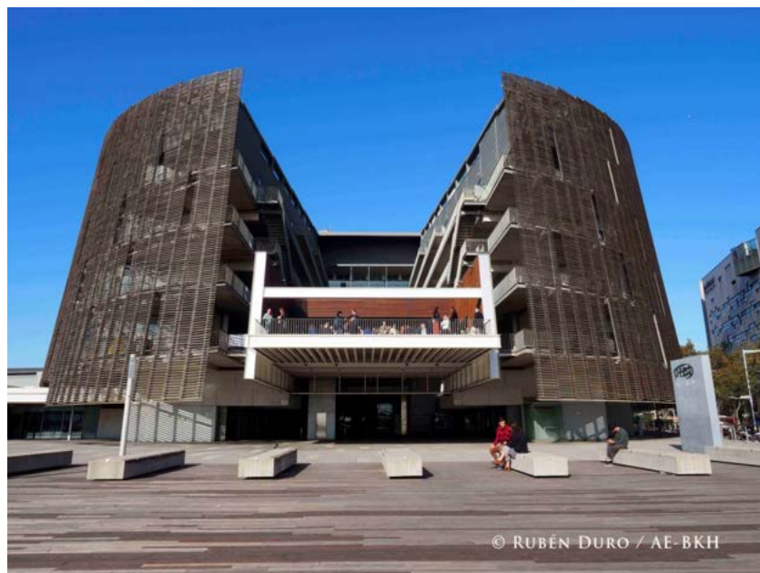
Two views of the PRBB Building.
